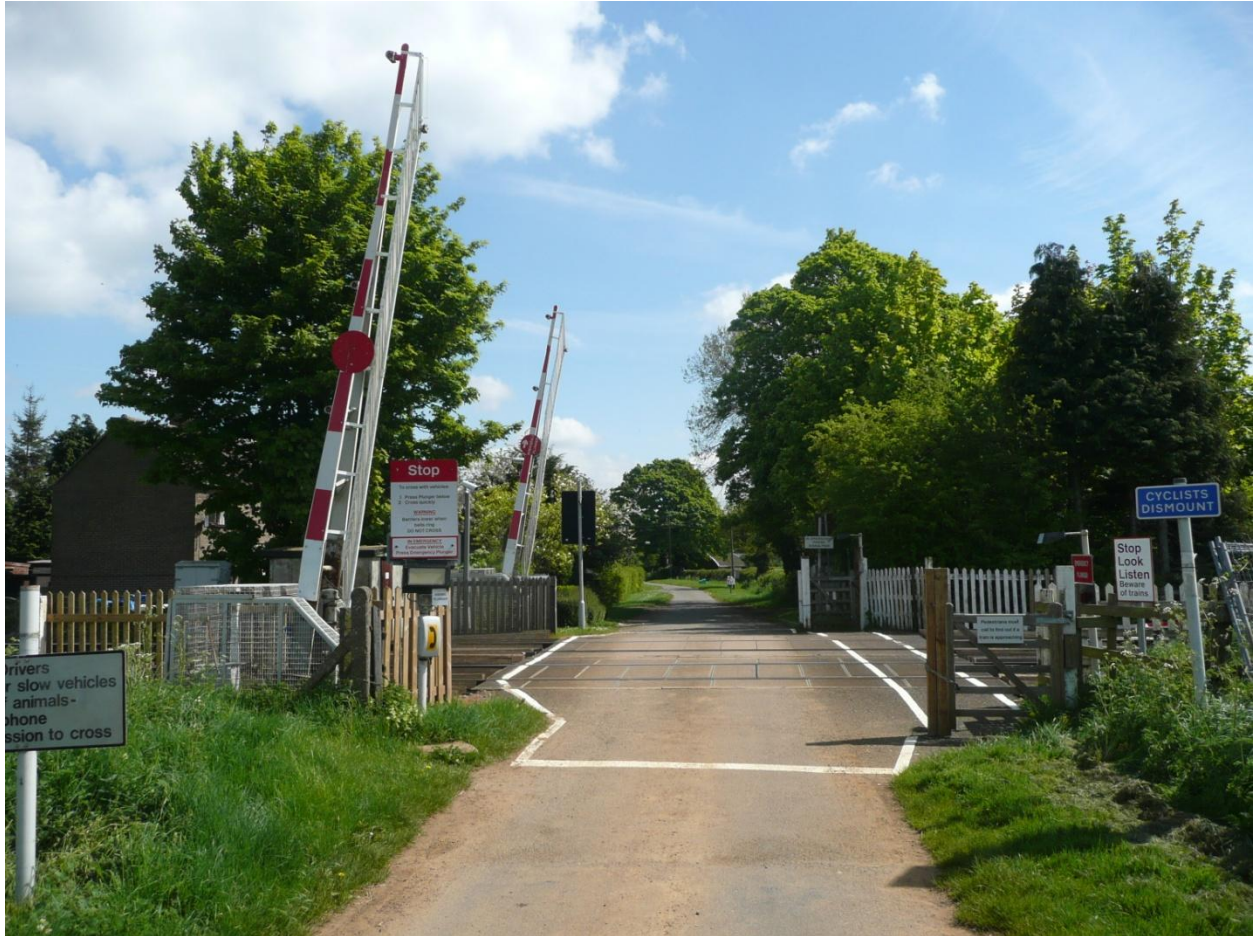
The Level Crossing at Ashwell
